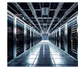
Designing the Next Era of Data Center Cooling: The Benefits of Modularization
