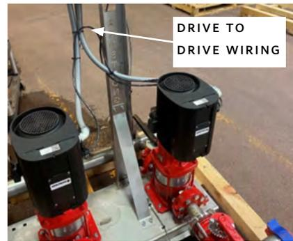
**4** Once the communications wiring is in the next drive, connect it to the wire harness as done in step 1.
